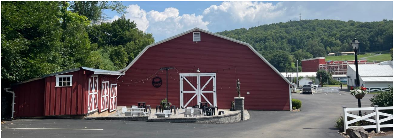
The historic Troy Sale Barn operated as a community livestock auction pavilion in the early 1920s and was slated to be torn down after years of non-use in 2014. Local citizens came together to purchase and restore the barn that is now used as a venue and community hall. (EMHR)
